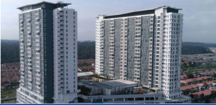
Figure 14: BSP Skypark (Bandar Saujana Putra, Selangor)
